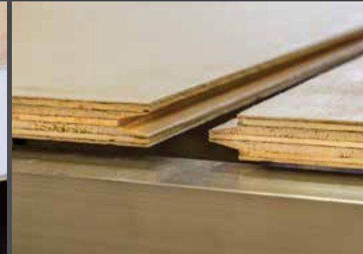
5/8" Tongue and Groove Plywood glued and screw to aluminum framing.
