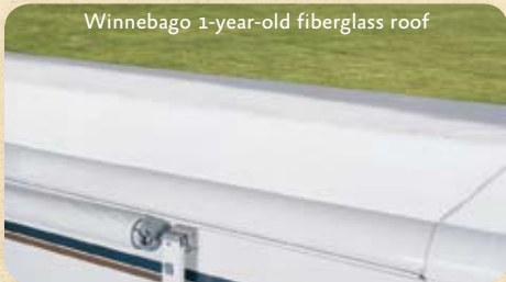
Winnebago 1-year-old fiberglass roof
