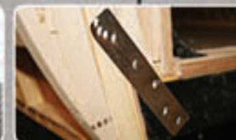
HURRICANE STRAP REINFORCED ROOF & WALLS
